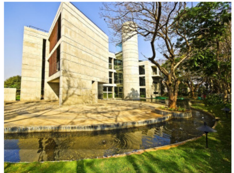
The reflecting pool that collects stormwater from the roof by SAMA Architects.
